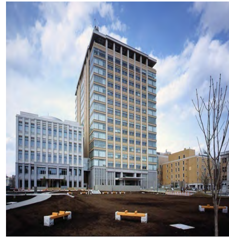
Tochigi Regional Government Building & Assembly Hall
