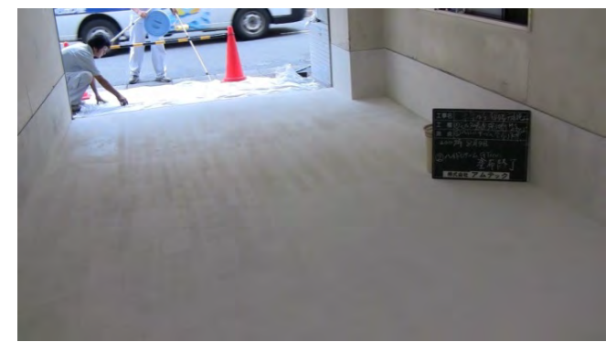
④ After Hydro-Dynam work
