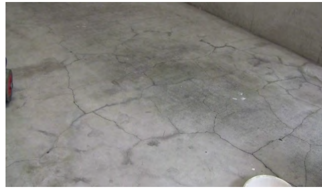
② Cracking on surface
